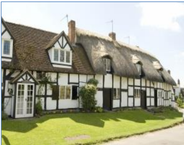
Figure 3 - Church Street (in the Conservation Area)
